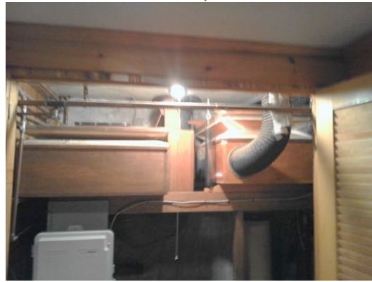
Blower and Reservoir, in basement directly below the organ:
