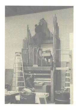
The proposal from Lewis & Hitchcock, Inc. was to rebuild the organ, keeping the original tonal plan, but using unit electro-pneumatic action for the manual windchests, to eliminate the problems of pneumatic duplexing, and rebuild the Gallery division into a true choral accompaniment organ.
