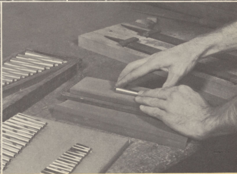
Final polishing of eschalots for reed pipes
