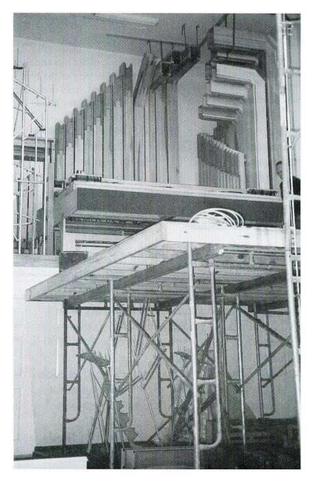
Behind the decorative cabinetry - The open wood pipes for the Grand and Pedal divisions of the instrument were among the first installed. These include the contrabasse, to the far right, which is 16 feet tall.
