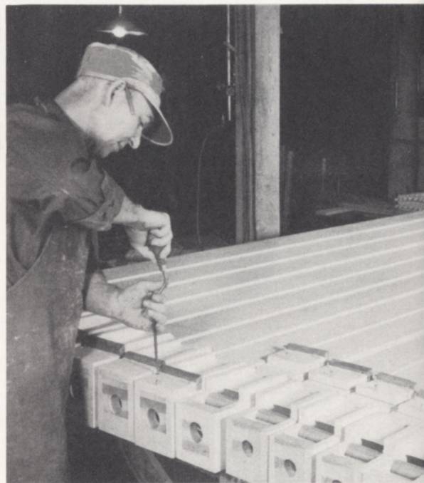
PRELIMINARY CUTTING OF THE UPPER LIP OF A WOOD PIPE
