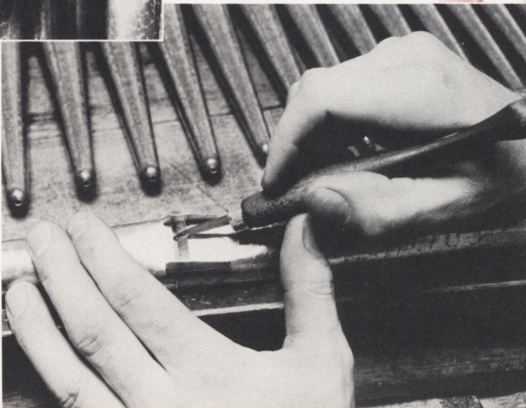
NICKING OR "CUTTING THE TEETH" IN A METAL PIPE
