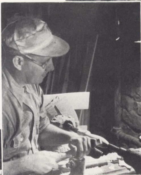
TURNING HANDLE FOR THE STOPPER OF A WOOD PIPE
