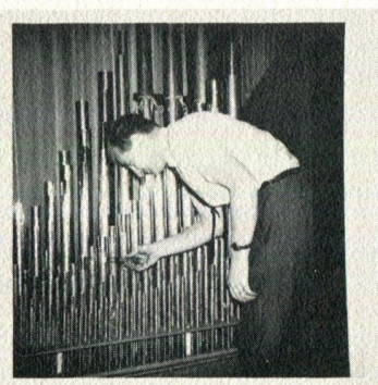
Regulating and tuning the pipes. Mr. Covell holding keys; Mr. Broome working on the pipes.
