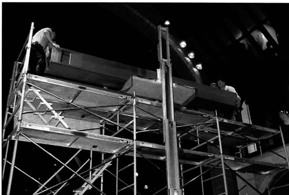
16' DIAPASON: Following shop restoration, each pipe (this one weighing approximately 300 pounds) was reinstalled into the organ chamber with the help of our hoist and 20 feet of scaffolding.
