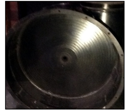
Inside of “sugar scoop” housing - before restoration
