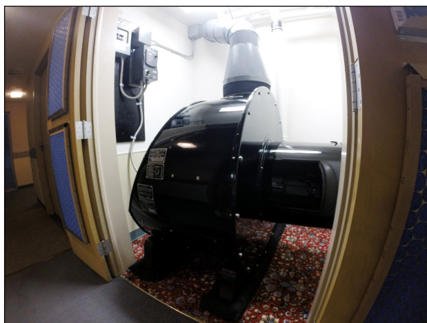
Assembled Orgoblo with new electric, wind line and new filter brackets on the blower room doors to help keep dust out of the organ.
