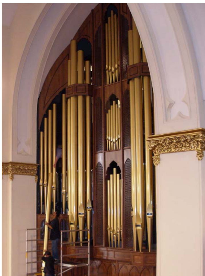
Installing façade pipes (photo credit Patty Conley)
