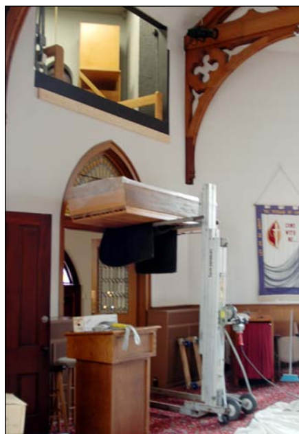
Hoisting the wind chest.
