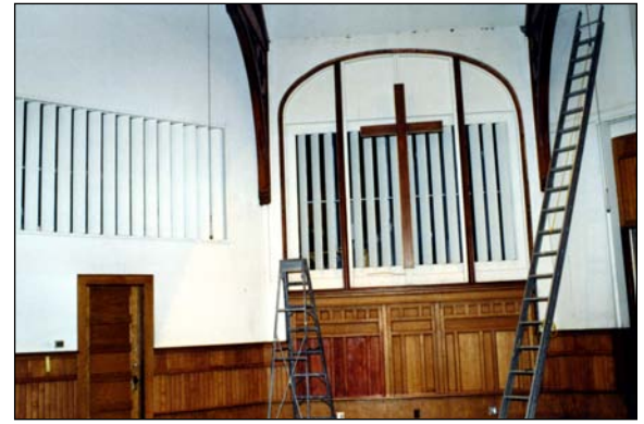
In 1995, the drapes were removed, revealing Swell shutters which control the volume of the organ. The Great division is behind cross and the Swell division is to the left.
