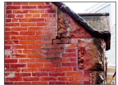
Areas missing mortar on church.
