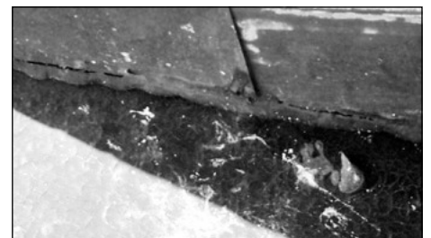
Failed flashing (2008).
